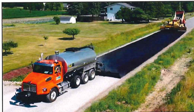
Iva Rd (Geddes & Frost) - Richland Twp Chip Seal
