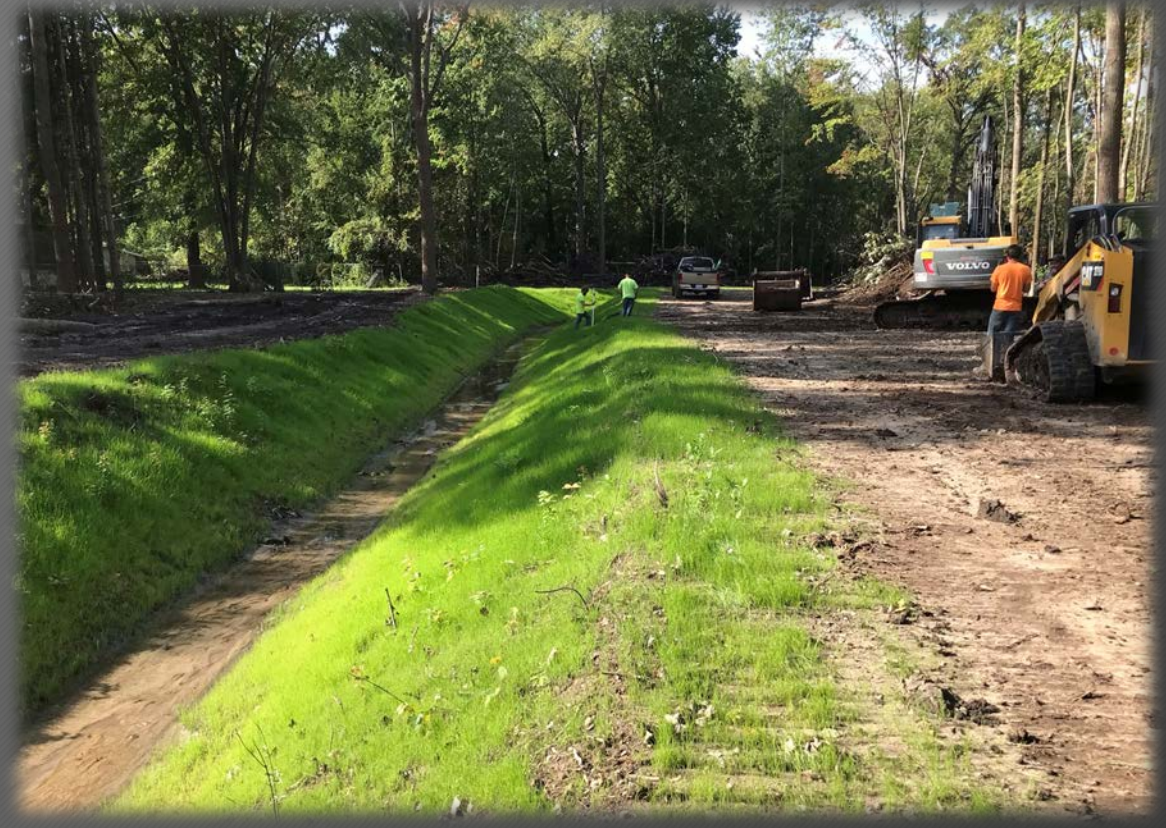
DRAIN AFTER CONSTRUCTION
